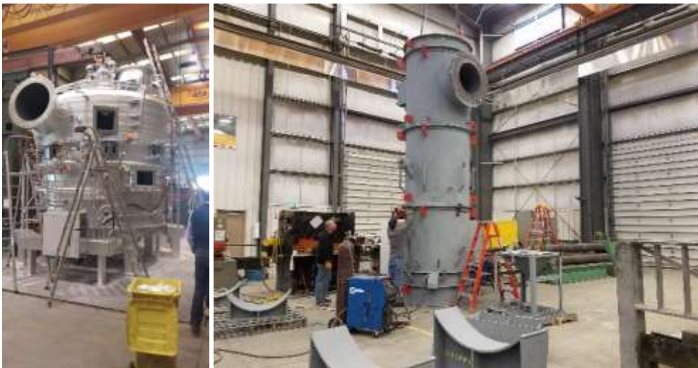
Equipment being installed at Commercial Demonstration Plant
