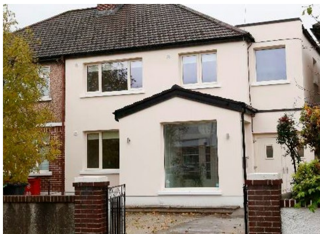
Figure 2.4: Before and after photo of 1960's home in Dublin that underwent a complete home energy upgrade under the SEAI One Stop Shop Service. Upgrade measures included external wall insulation, floor and attic insulation, triple glazed windows, and heat pump installation. The project was completed by KORE Retrofit, a registered One Stop Shop provider under the scheme. (Copyright: KORE Retrofit, 2023)
